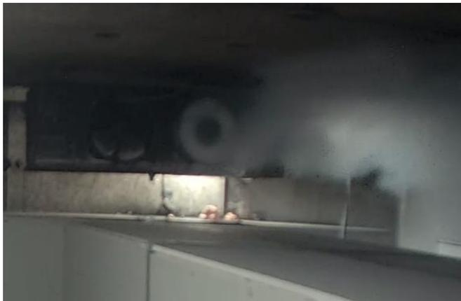
The discharge in the coil face caused the fan to rotate. Note the frost buildup on the right-hand fan blades.
