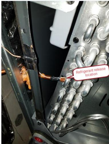
Refrigerant release location for leakage in A-Coil Scenario
