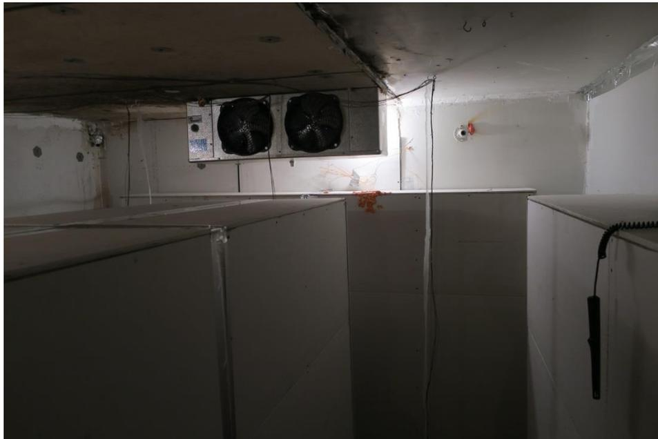
Figure 126 - Camera view of evaporator mounting and obstructions
