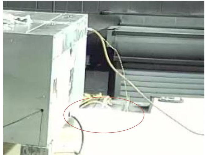
Condensate Drain on RTU showing a mist escaping through this route. The power cable for the fan motor was routed through the condensate drain.
