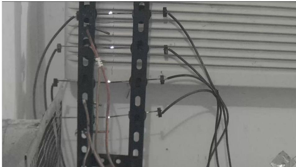
**Figure 103 – Electric arcs and refrigerant sampling tubes immediately in front of discharge location**
