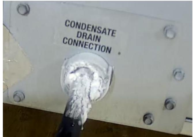
Condensate Drain on RTU showing maximum ice build up and condensation escaping through this route. The power cable for the fan motor was routed through the condensate drain.
