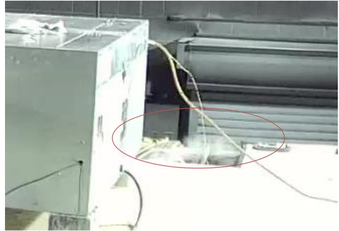
Condensate Drain on RTU showing a mist escaping through this route. The power cable for the fan motor was routed through the condensate drain.
