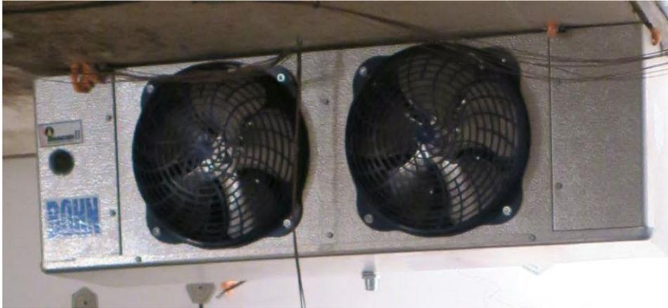
Figure 173 – Walk-in Unit Cooler
