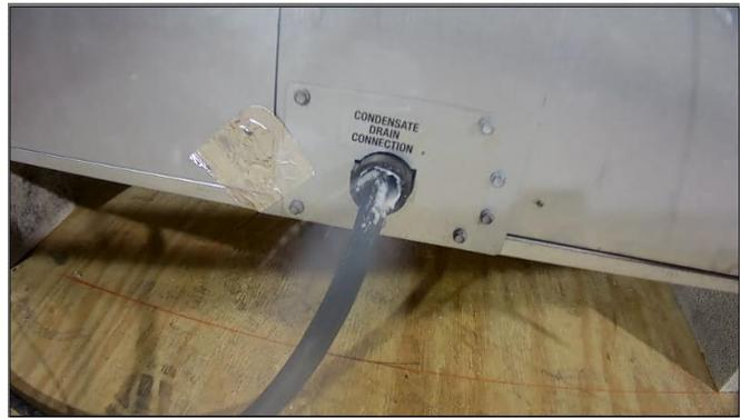
Condensate Drain on RTU
