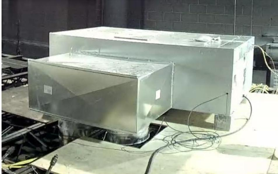
**Figure 114 – Roof top unit (supply side)**
