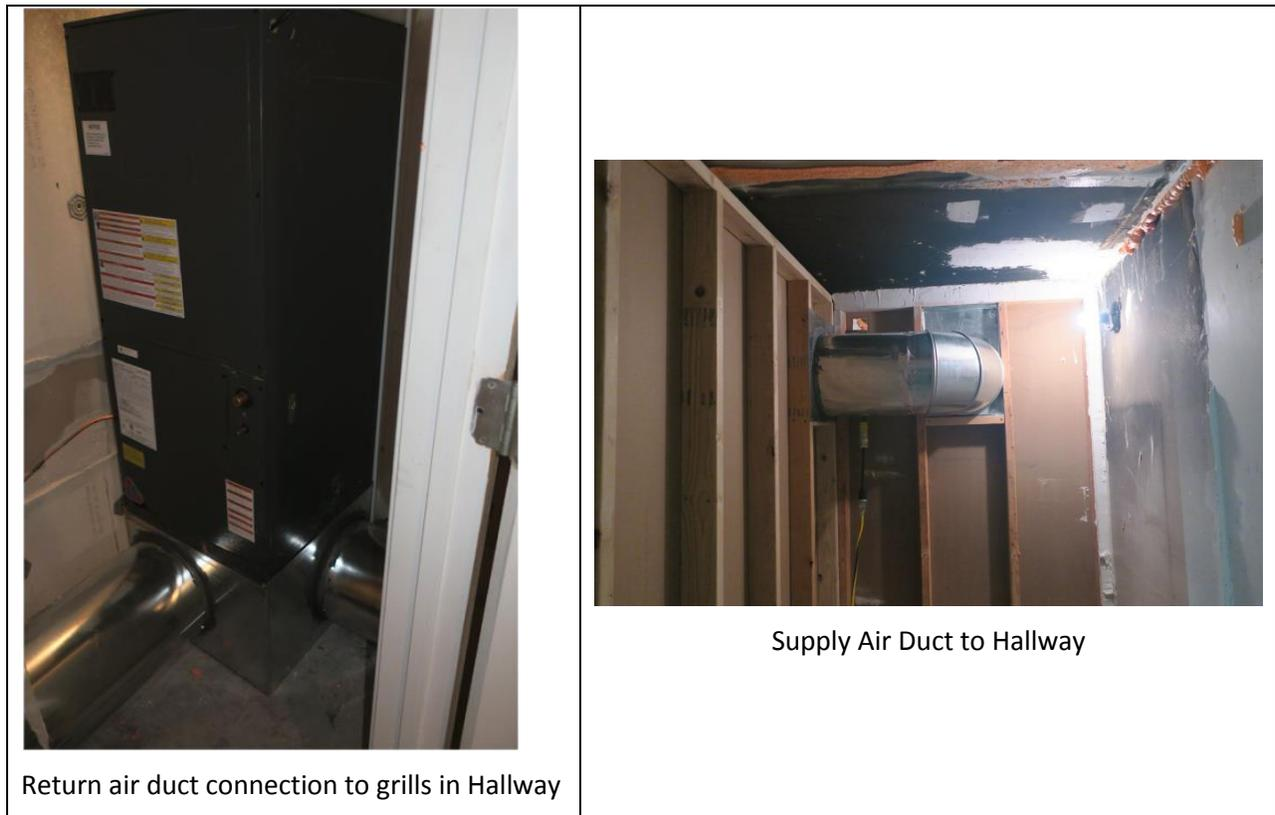
**Figure 136 – Return Air and Supply Ducts Air connecting to Air Conditioning Unit**
