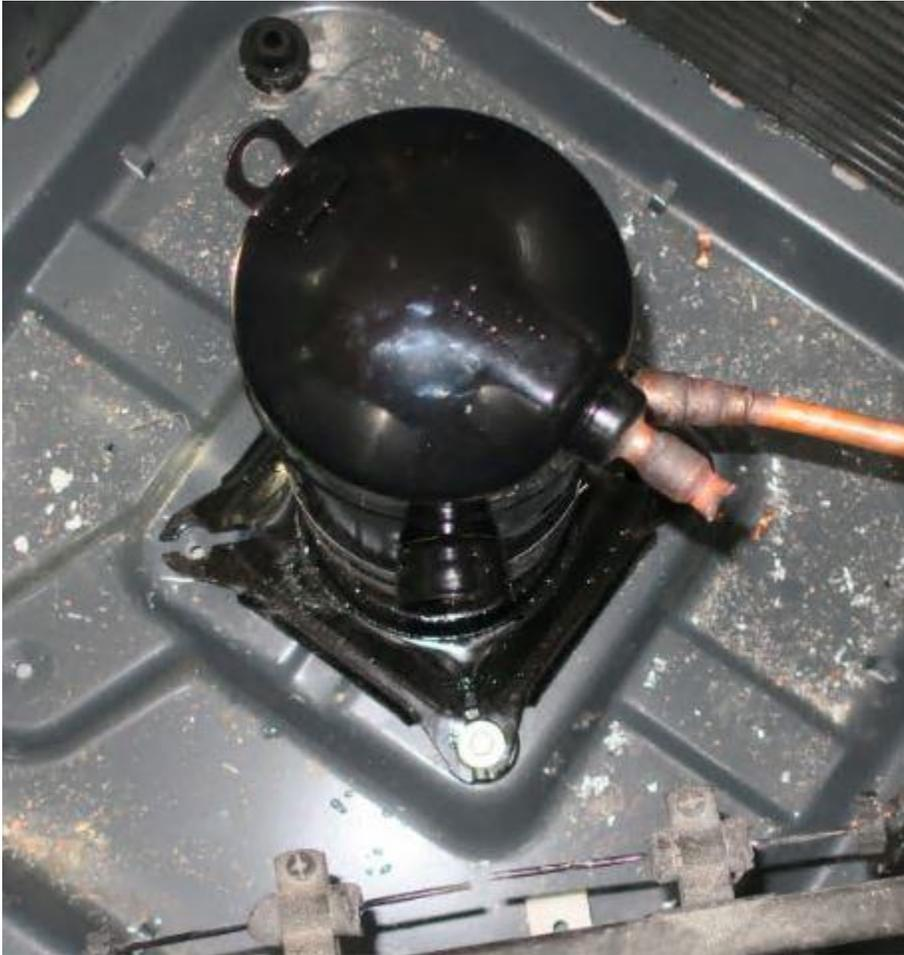
Figure 171 – Outdoor Compressor (Hermetic Electrical Pass-Through Terminal Failure Tests)
