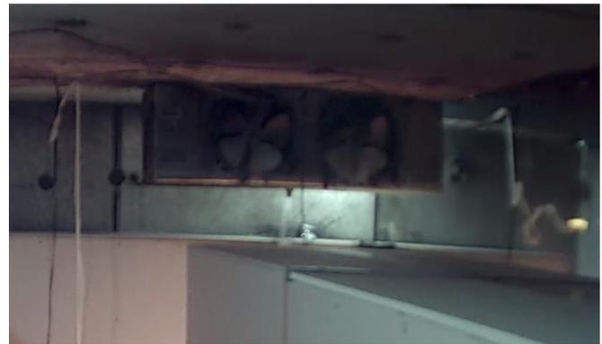
It appears that liquid refrigerant is dripping from the drain at 63 seconds after the start of the discharge.
