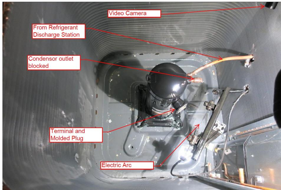
**Figure 150 – Interior Arrangement of Condensing Unit Components**
